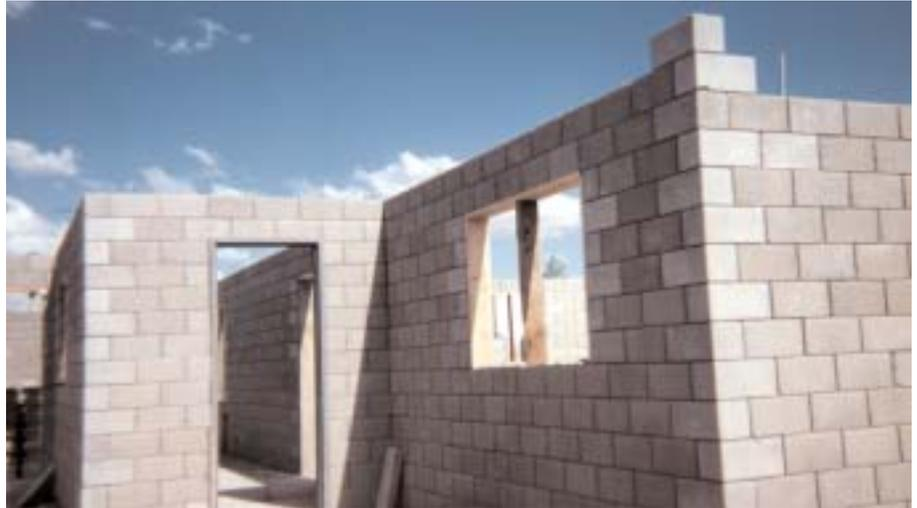
The Haener Mortarless Interlocking Block is a modular system which is dry stacked in running bond without mortar and then filled with grout to provide a finished wall.
